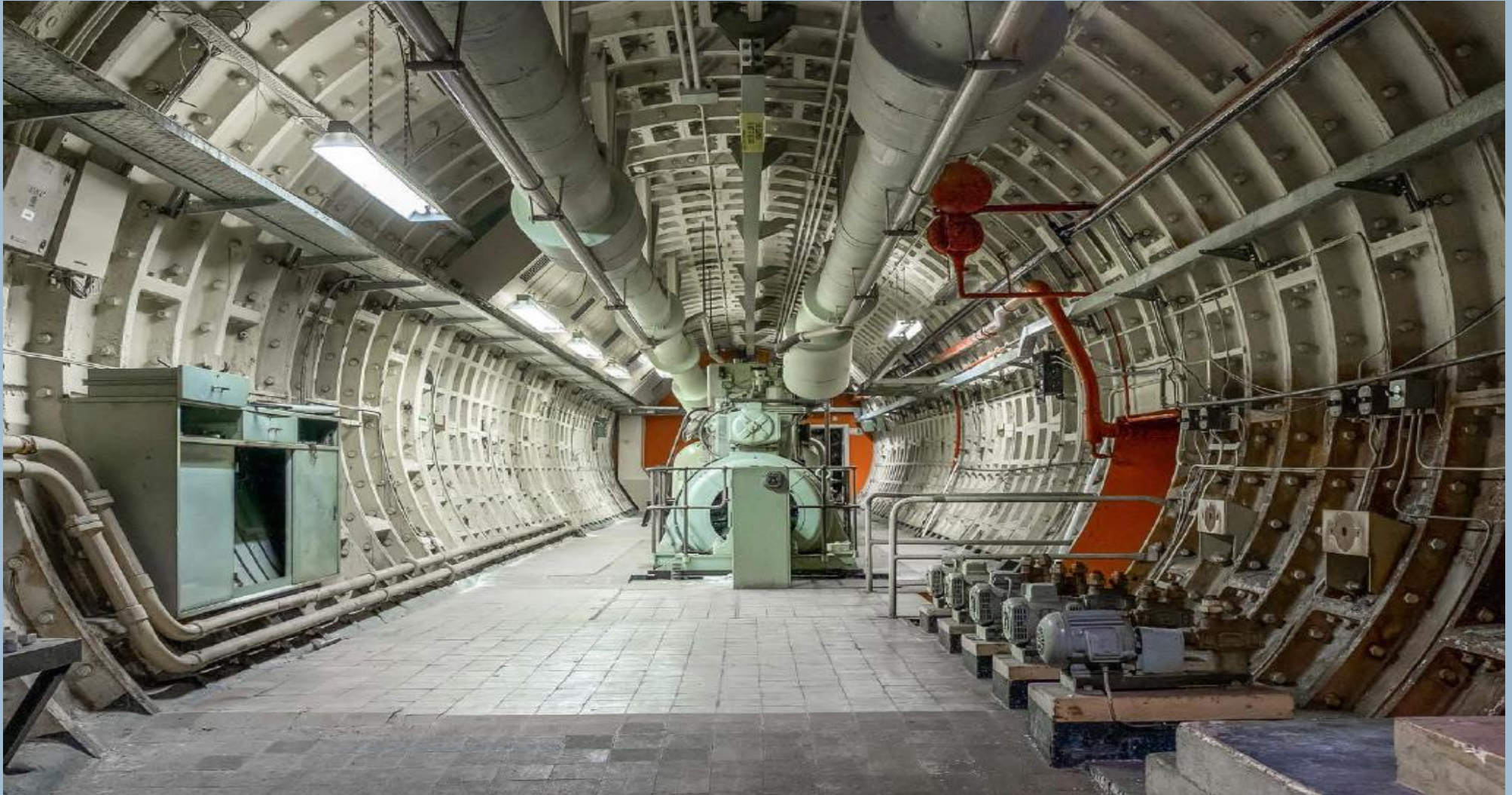
Inside one of the smaller tunnels | 5.5m diameter.
