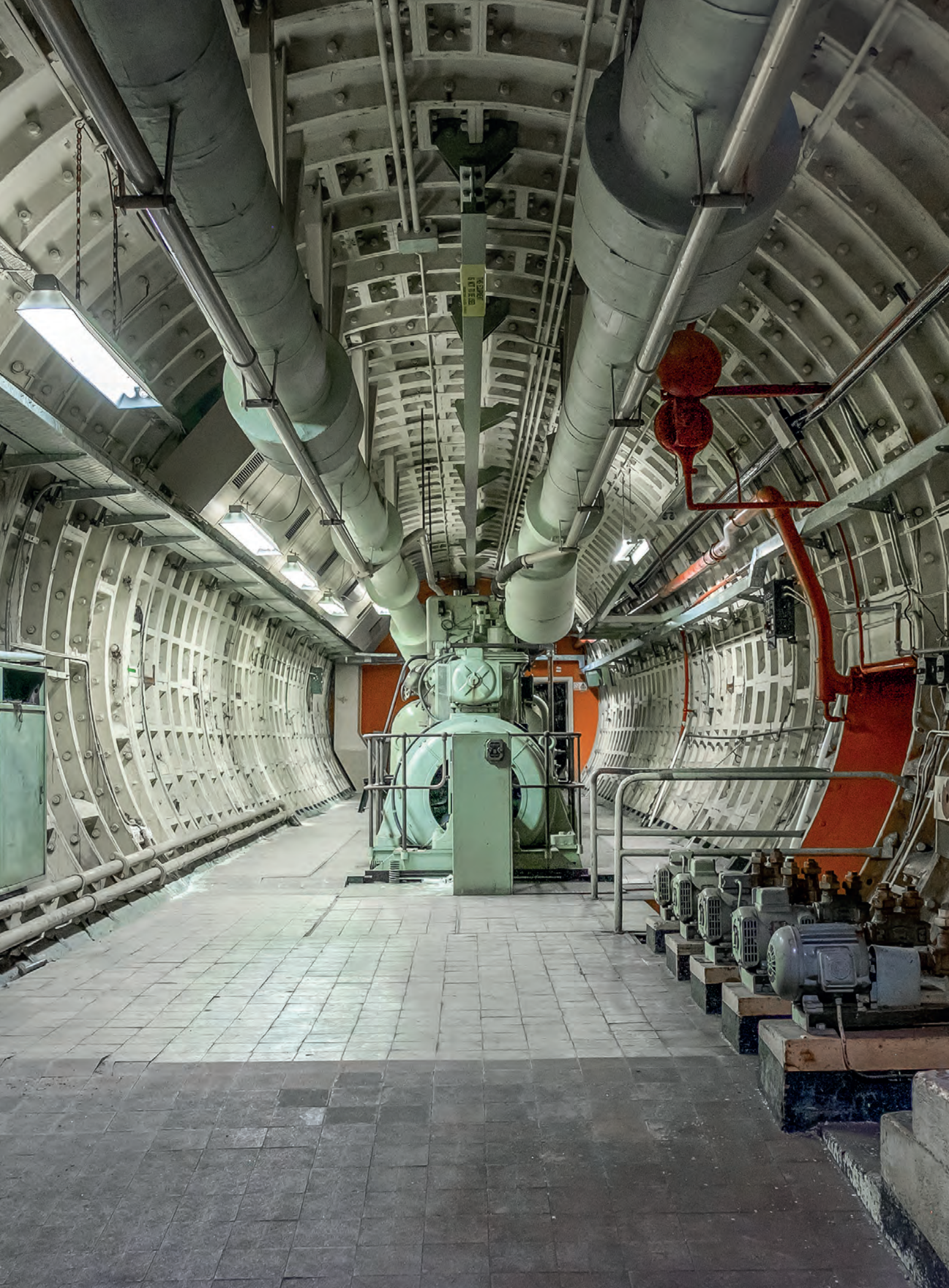
A snapshot of the Tunnels in their current state
