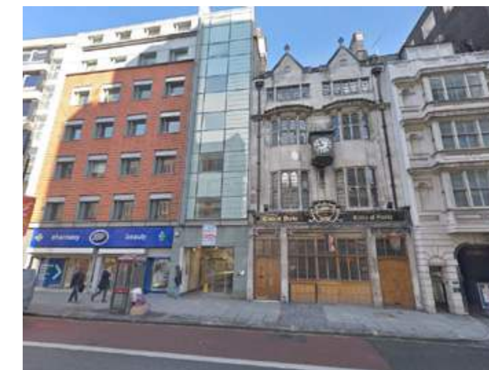
Poor quality piecemeal development leading to erosion of historic character and identity
