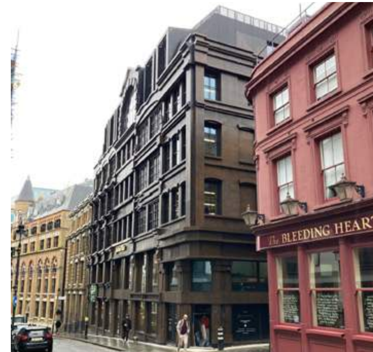
28 Greville Street, office refurbishment in Hatton Garden
