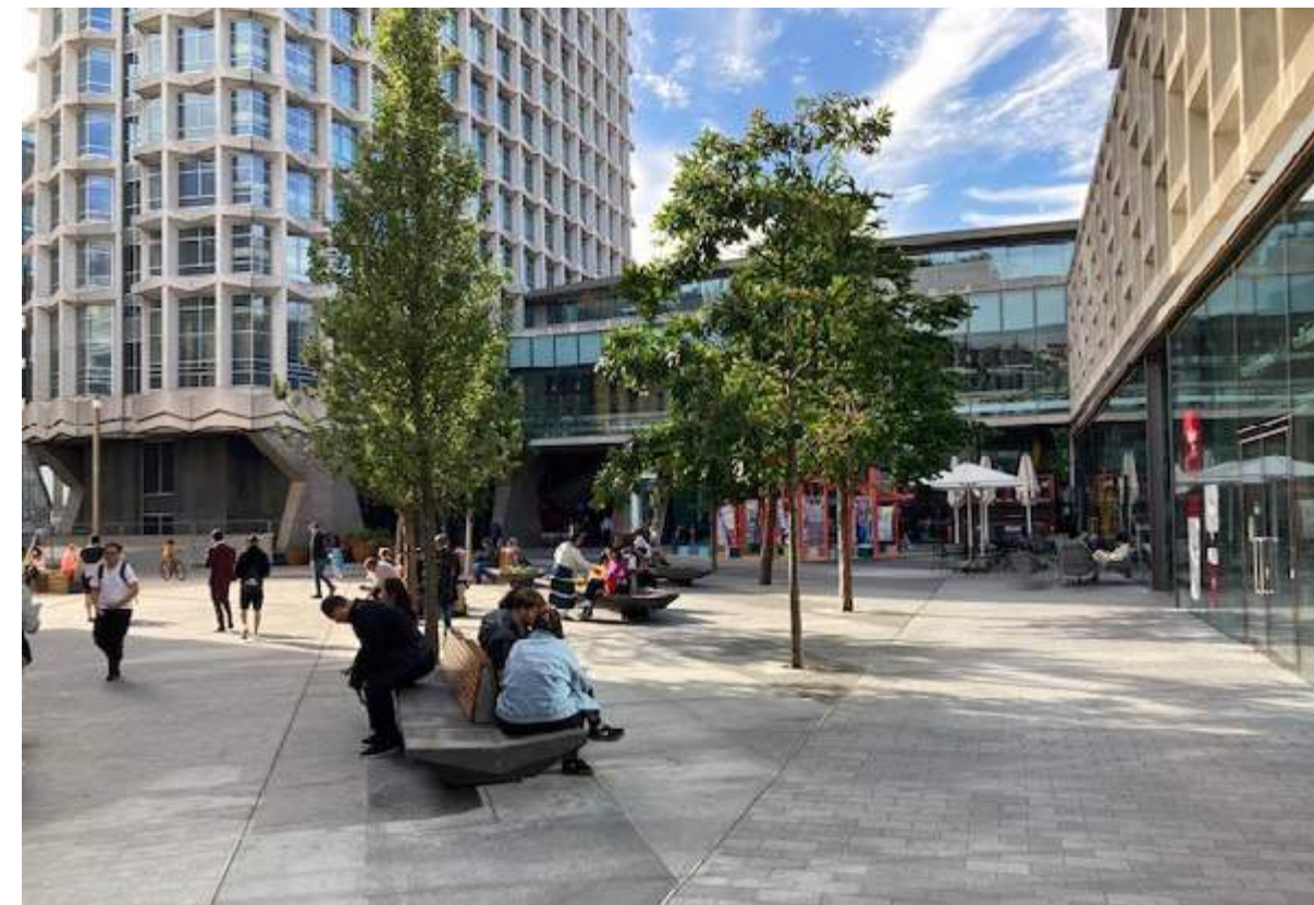
Centre Point and St Giles Square, recently completed
