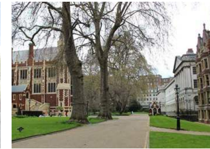
Older building stock has lower EPC scoring - Lincoln's Inn Fields example (image from LDA report)
