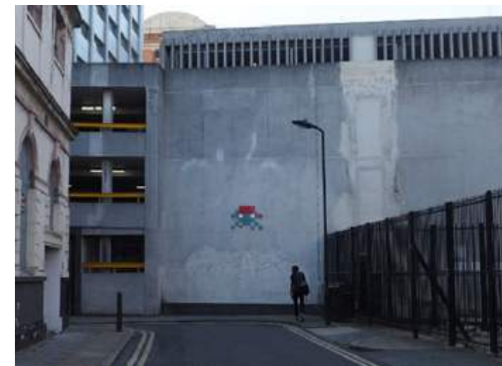
Inactive frontages and a lack of permeability
