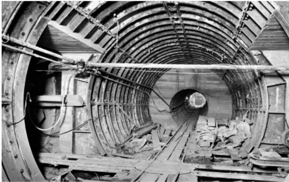
Air raid shelters were ordered after the start of the bombing raids on London. DBOX/The London Tunnels
